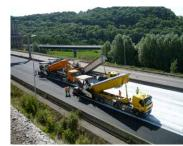
Asphalt laying after Asphacal®TC spreading
